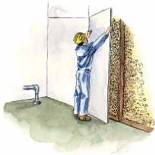
Protect installed foam with a thermal barrier such as  $\frac{1}{2}$ " gypsum board as soon as possible
